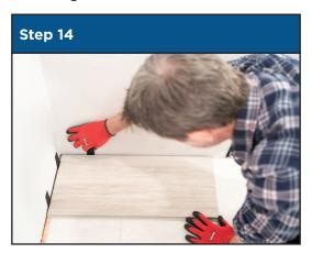
Fig. 1: Use guide tile to lock in fourth tile.
